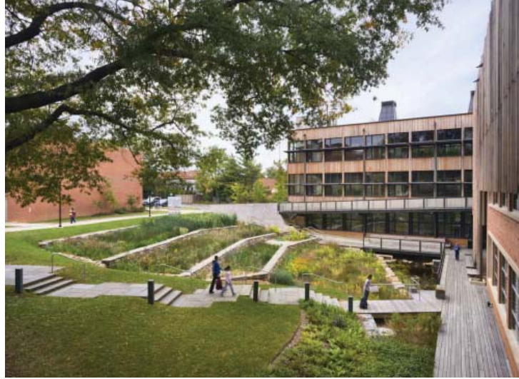
sidwell friends middle school, dc (kieran timberlake associates)
