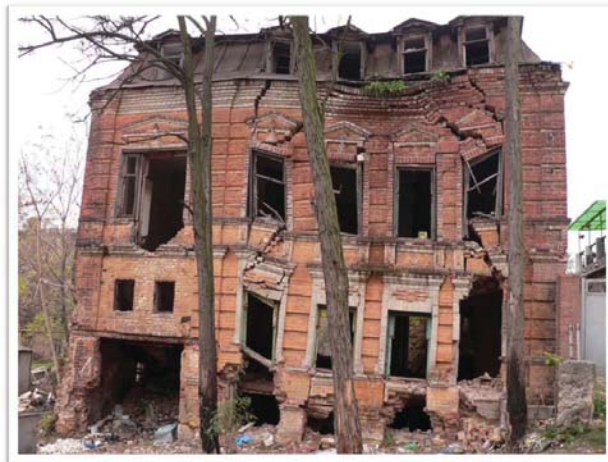
Buildings can...and will fail when not properly taken care of.
