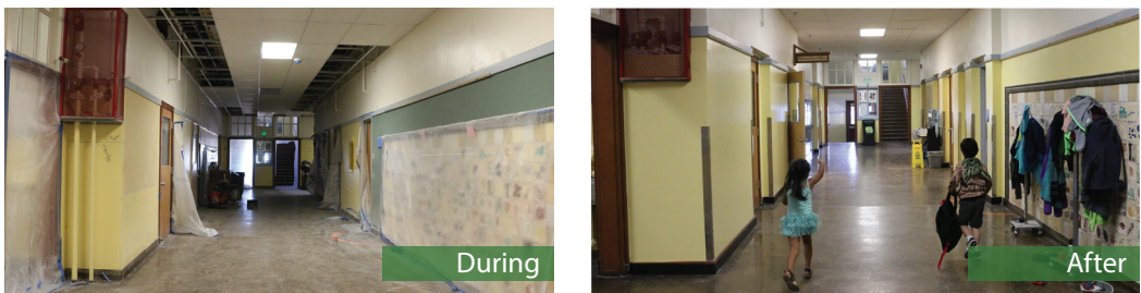
Seismic bracing of hollow clay tile in the main hallways.
