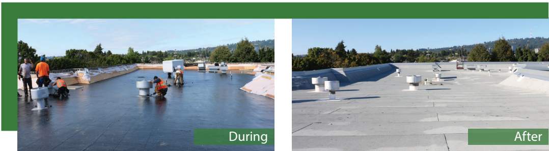
Roof level seismic improvements with re-roofing that will include new insulation, some rooftop mechanical, roofing materials and roof ladders.
