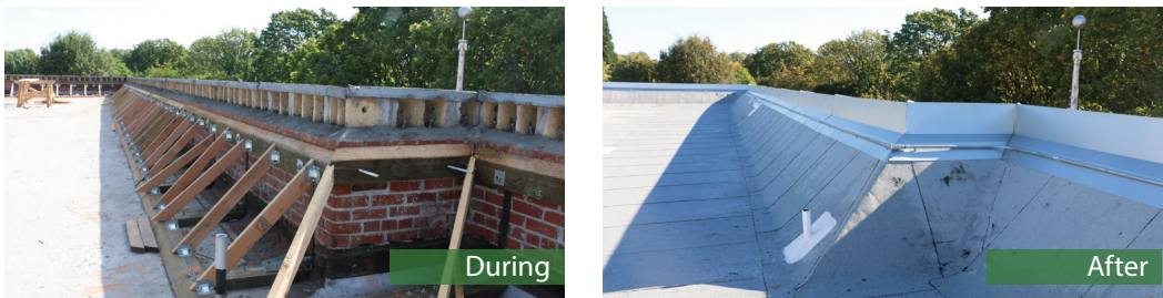
Roof level seismic improvements with re-roofing that will include new insulation, some rooftop mechanical, roofing materials and roof ladders.
