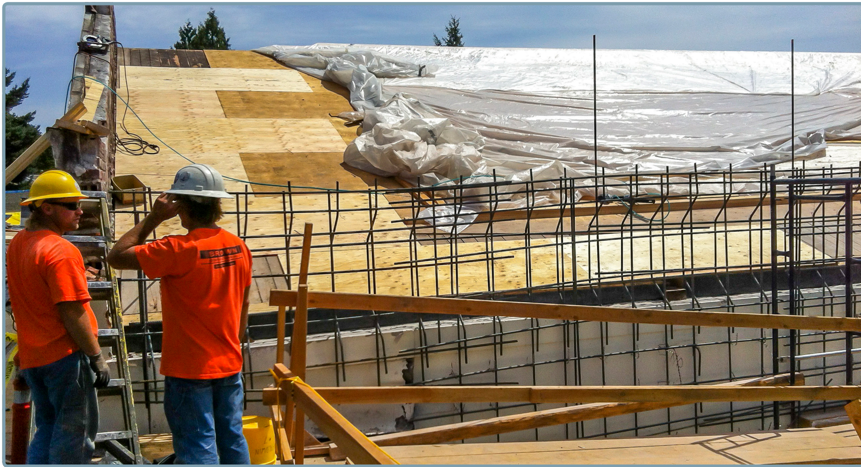
Complete roof replacement with seismic strengthening, new skylights and mechanical equipment added
