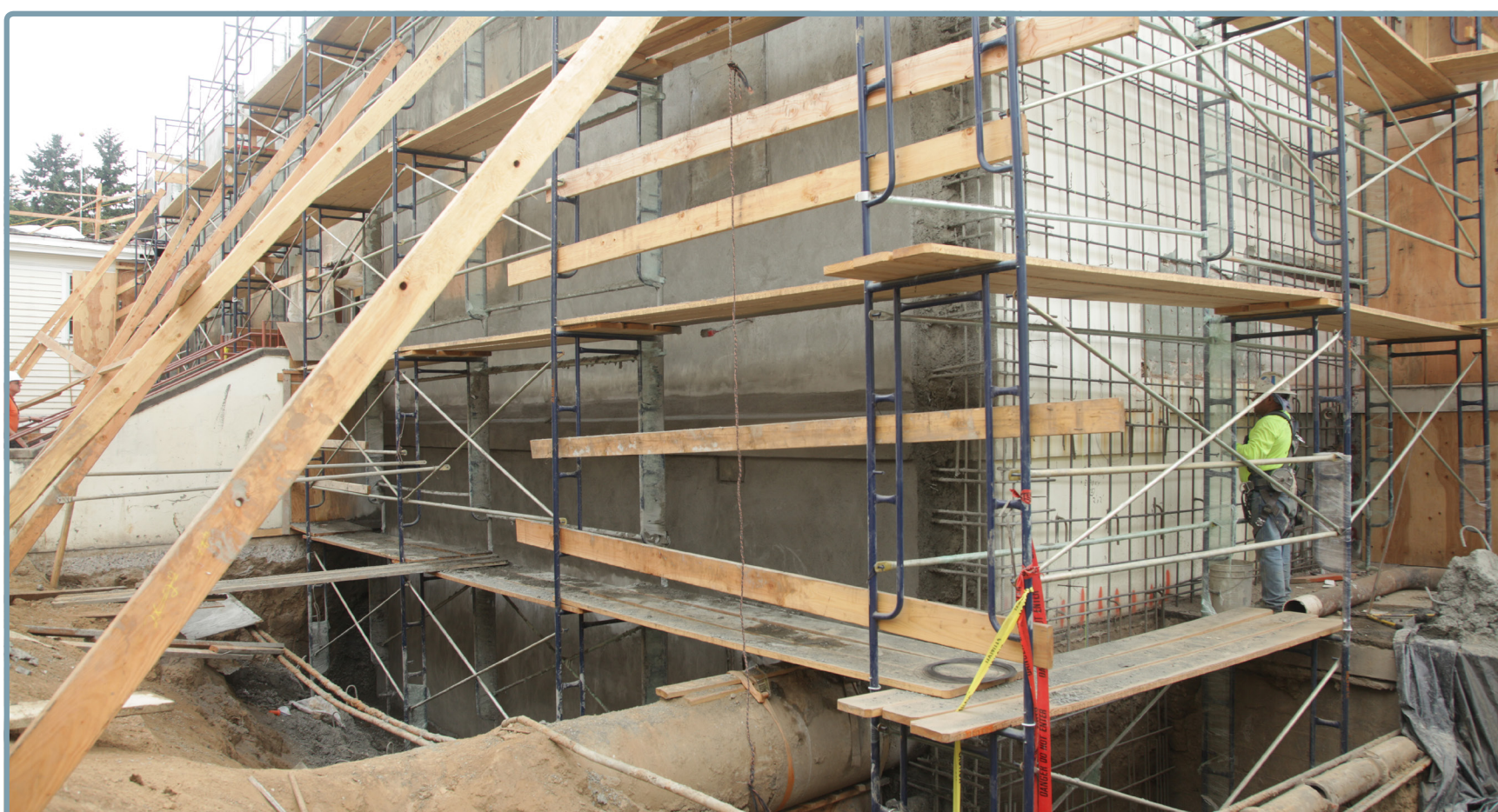
Seismic strengthening of the cafetorium
