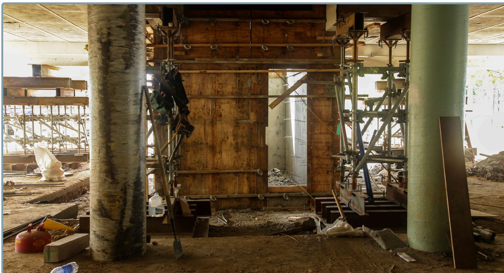
Seismic strengthening of the 1953 addition
