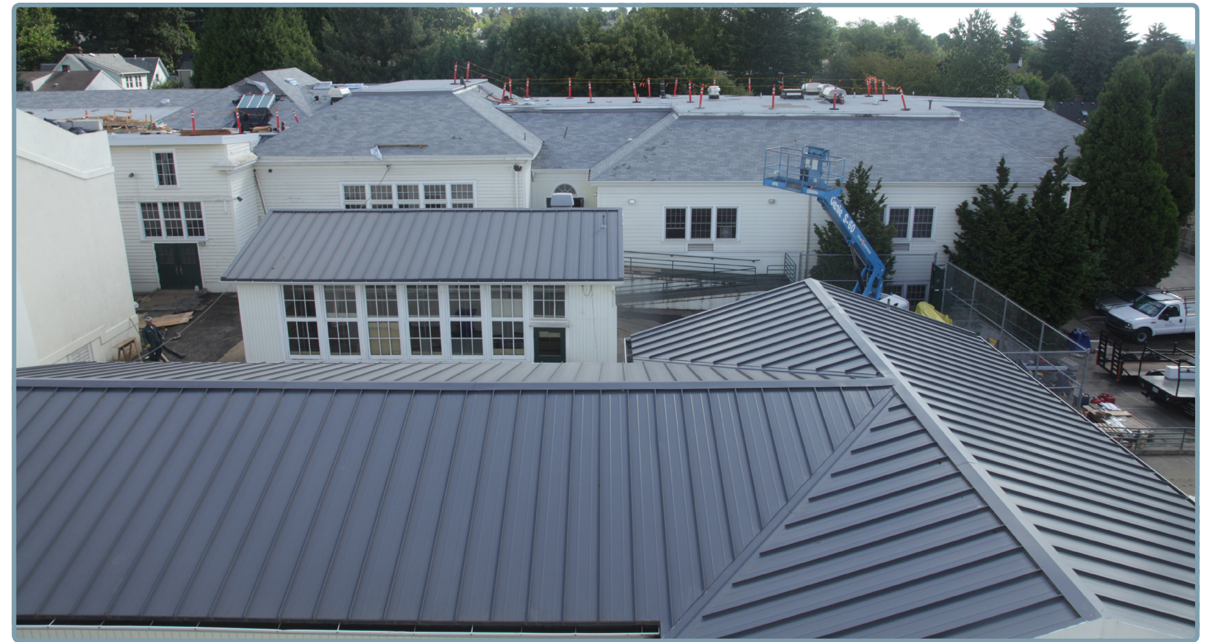
Complete roof replacement with seismic strengthening, new skylights and mechanical equipment added
