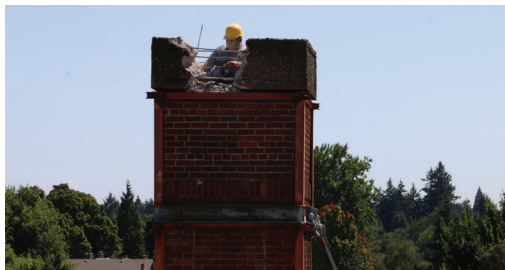
Removal of the brick chimney.
