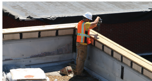
Roof level seismic improvements with re-roofing that will include new insulation, rooftop mechanical, roofing materials, roof ladders and new steel trusses in the gym penthouse.
