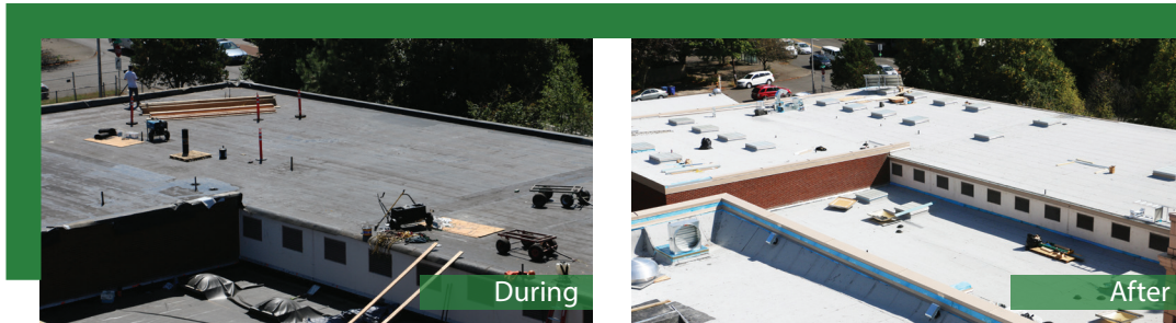
Roof level seismic improvements with re-roofing that will include new insulation, rooftop mechanical, roofing materials, roof ladders and new steel trusses in the gym penthouse.
