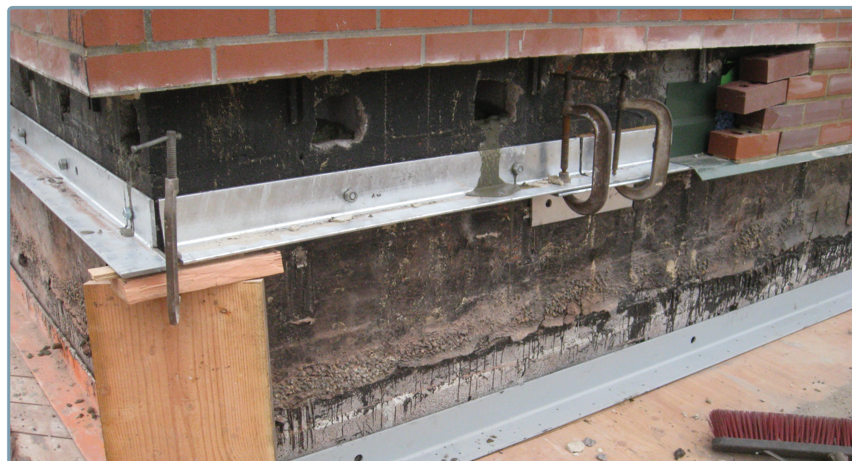
Removing the old roof materials and installing roof-level seismic upgrades.
