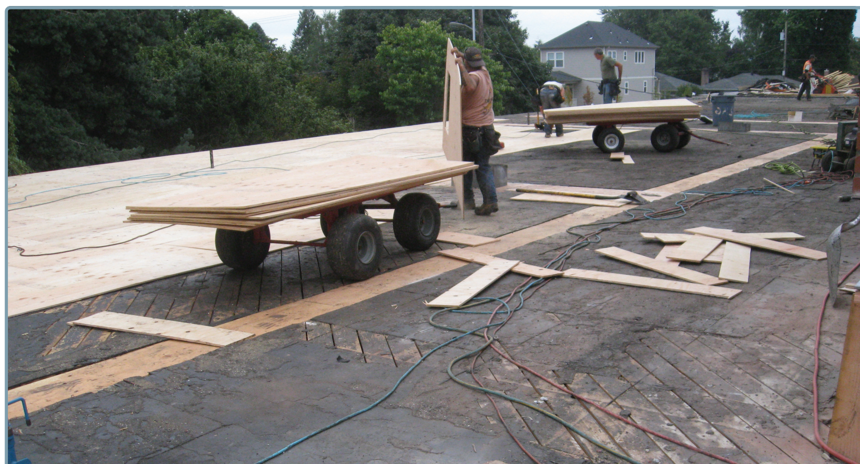
Removing the old roof materials and installing roof-level seismic upgrades.
