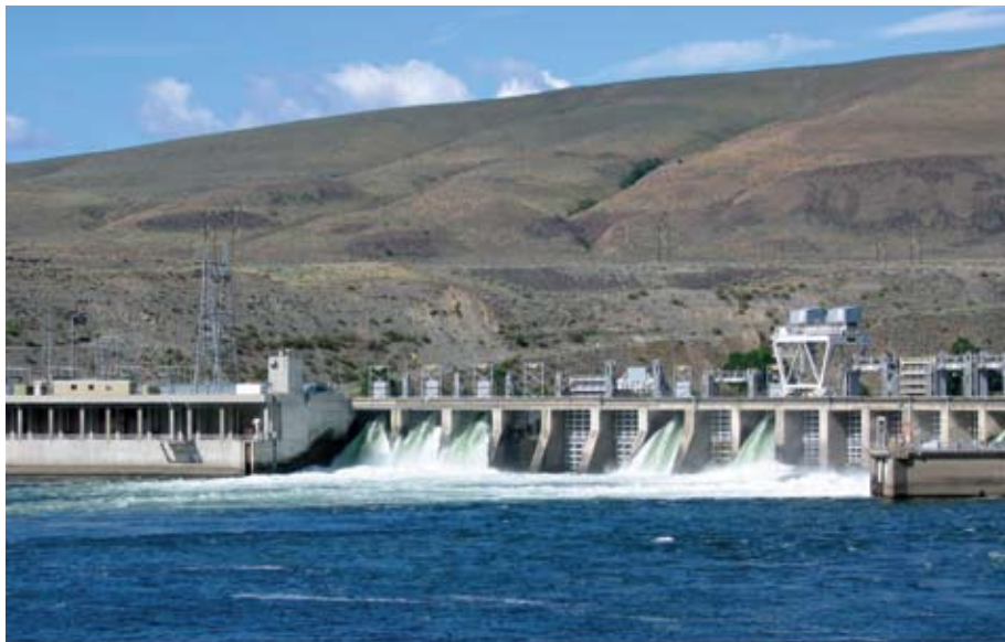
Hydroelectric dam in the Northwest
