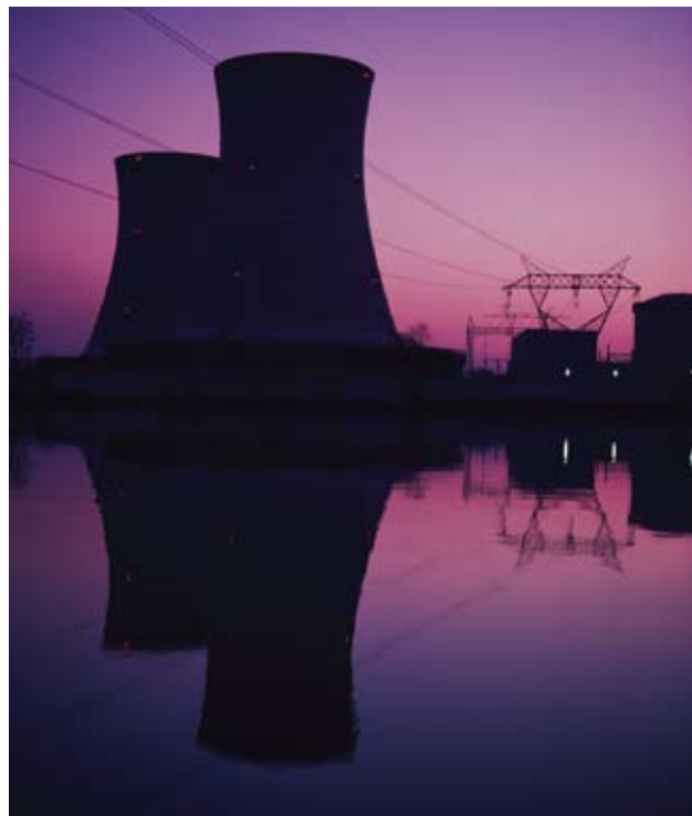
Nuclear, coal, and natural gas power plants require large amounts of water for cooling. 191
