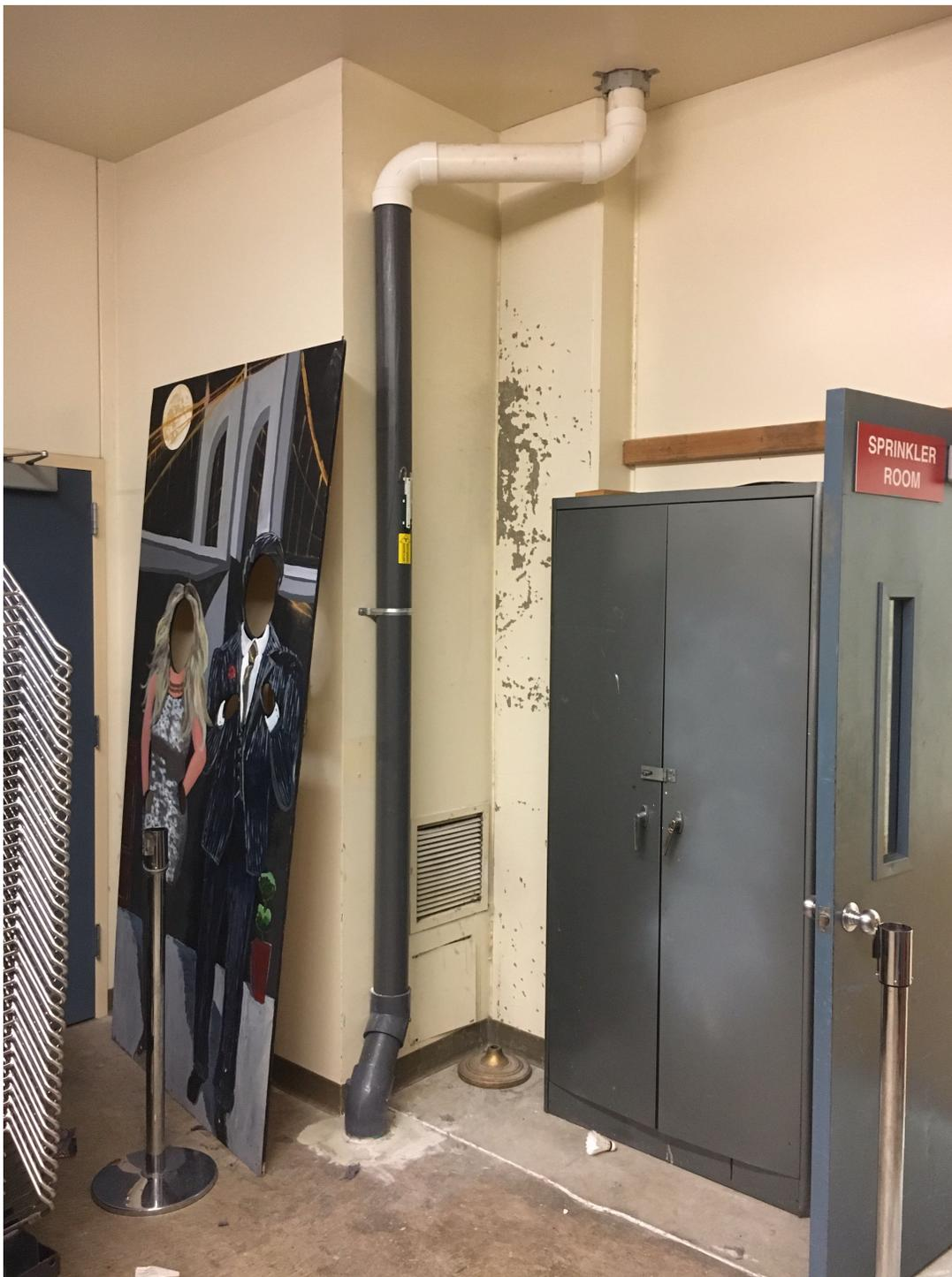
**The suction point is located in a storage room adjacent to the gym. The vent piping continues to the mechanical room above and then to fan location on the roof. The system includes a manometer (pressure gauge), which is a simple means of seeing the system is working mechanically. A manometer also shows how much negative pressure (depressurization) the system is creating. It is understood such a pressure gauge DOES NOT monitor radon levels.**
