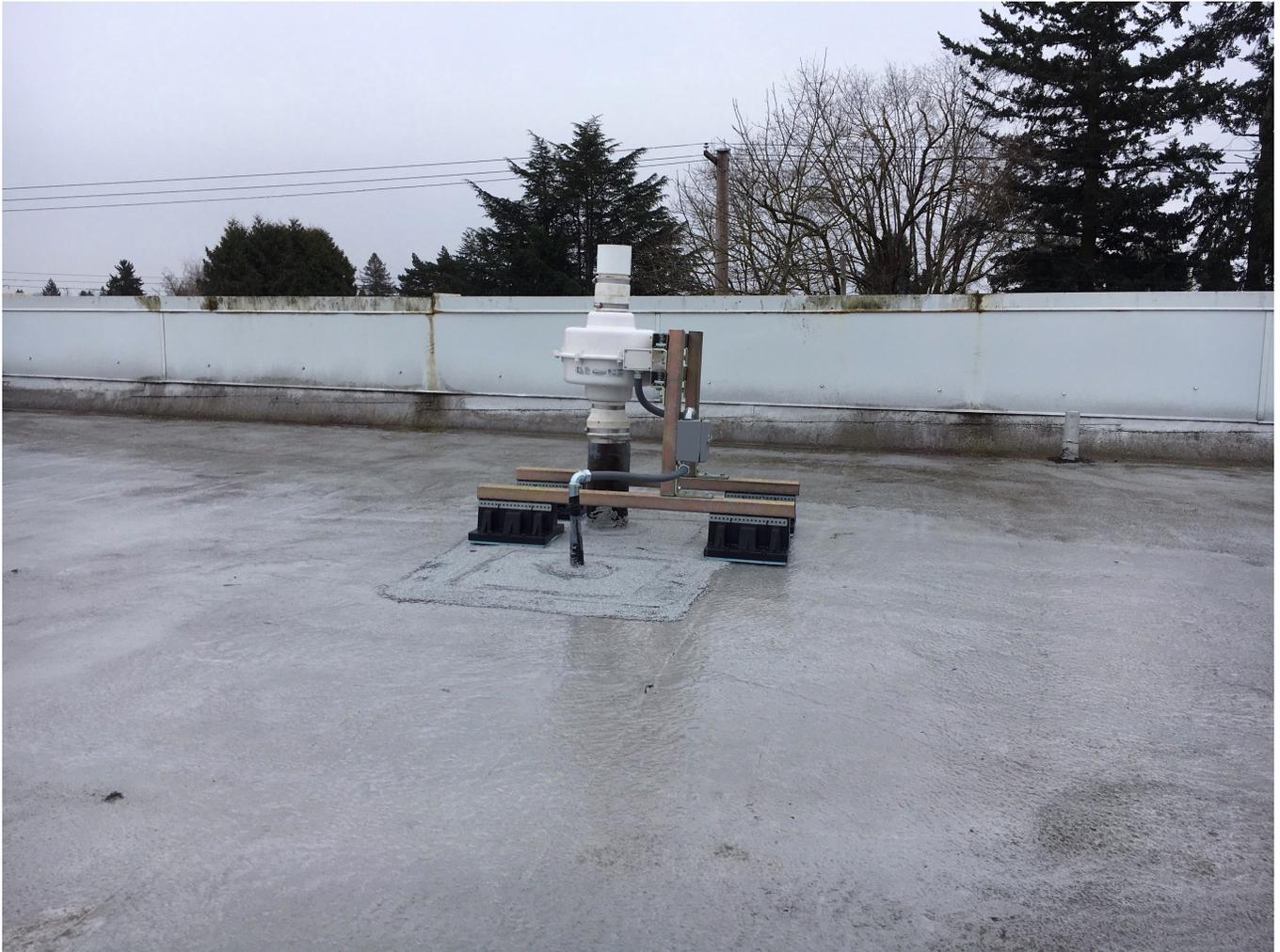
**This system required a RadonAway GP501 model fan, which is designed for the denser soil found beneath the concrete slab. For secure and durable mounting, a strut channel stand was constructed to support the fan and electrical components. If left to operate continuously the lifespan of this fan typically is 10 to 15 years.**
