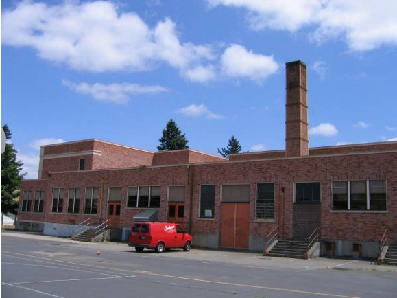
West elevation facing east
