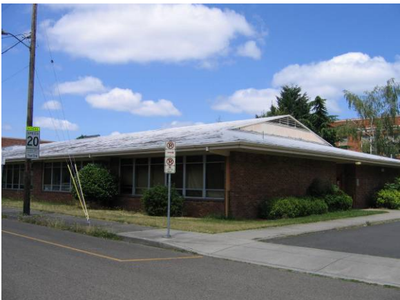
Annex looking northwest
