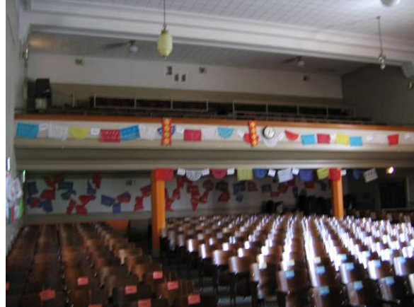
Auditorium facing west
