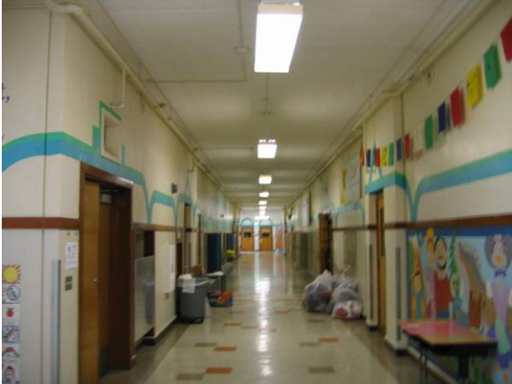
Corridor facing north
