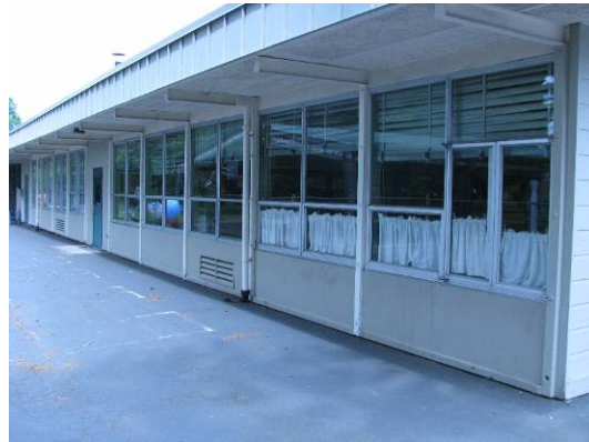
Bank of windows located on south elevation (256A).
