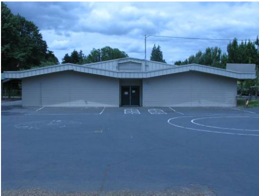
East elevation entrance (256A).
