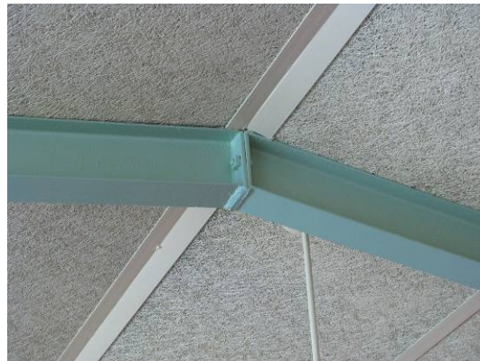
Detail of ceiling beam (256A).
