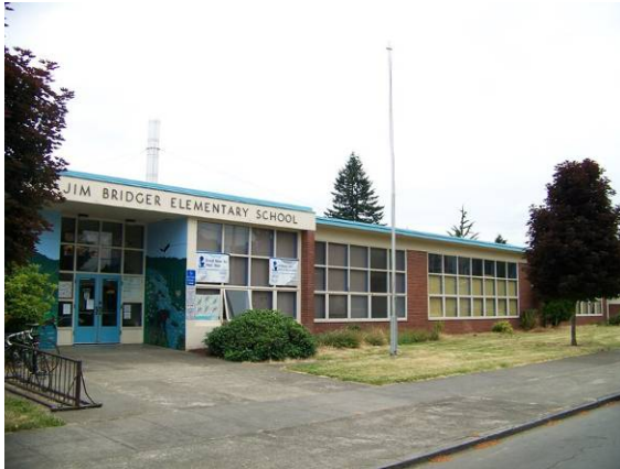
Main building (238A), north (front) elevation looking south.
