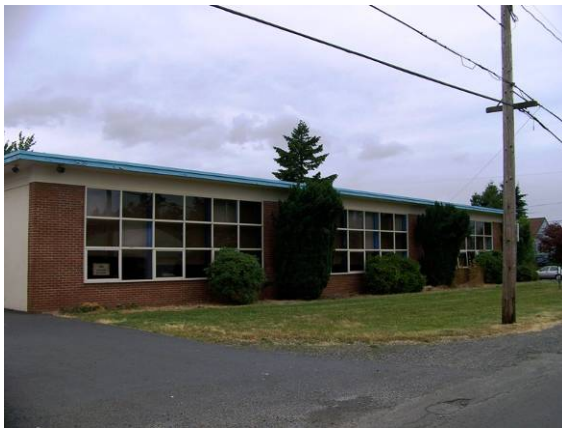
Main building (238A), east (side) elevation looking northwest.
