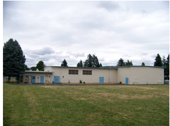
1959 Addition (238A), west (side) elevation, looking east.
