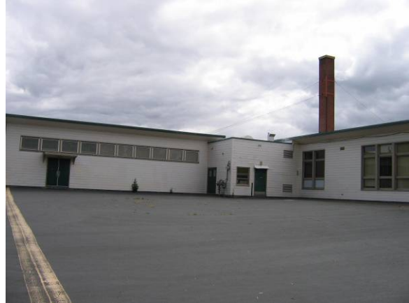
South elevation looking north
