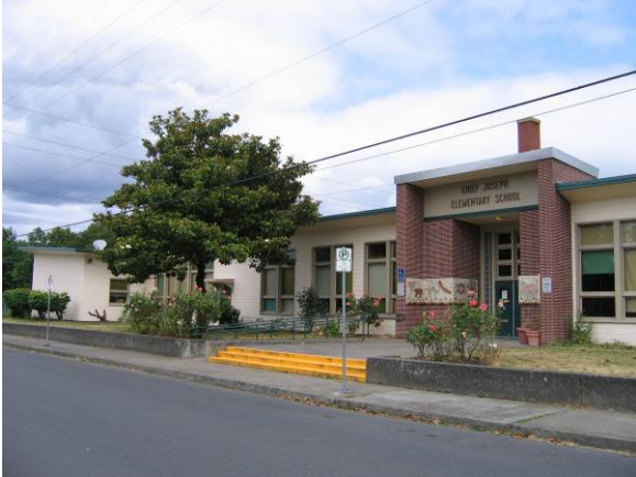
South elevation facing northeast
