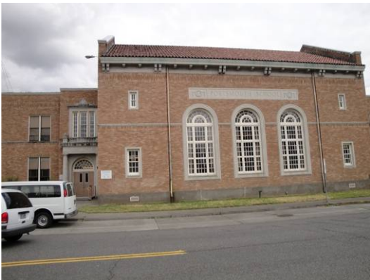
South elevation front entry (and auditorium)
