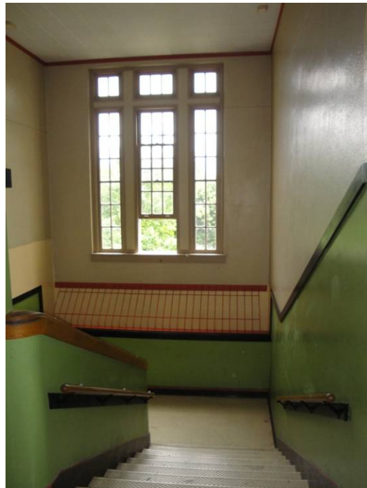
Stairwell facing south
