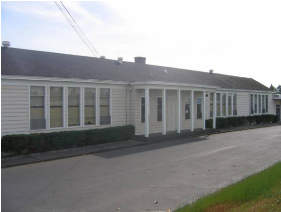
East elevation facing northwest
