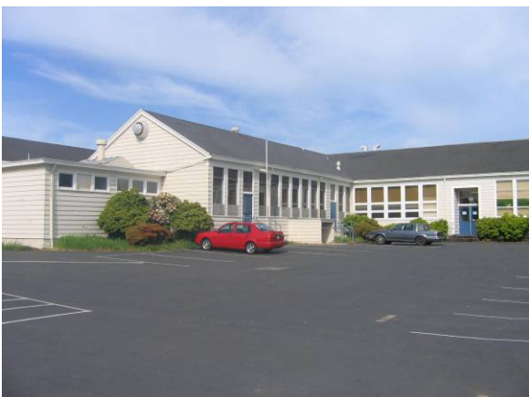
West elevation facing east
