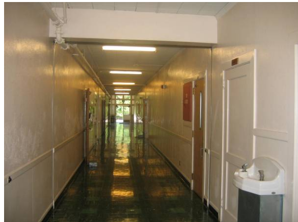
Corridor facing east
