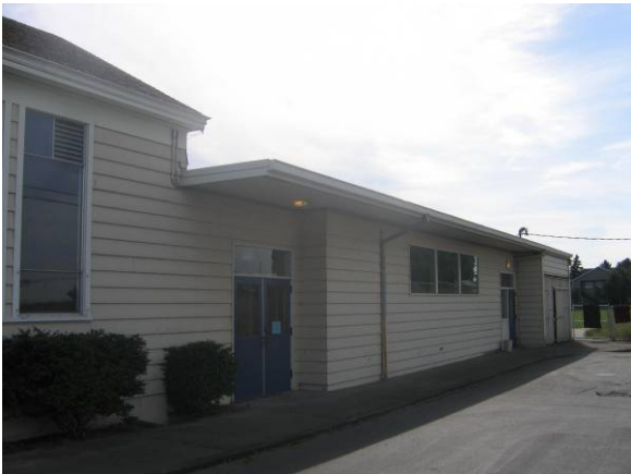
North elevation facing south
