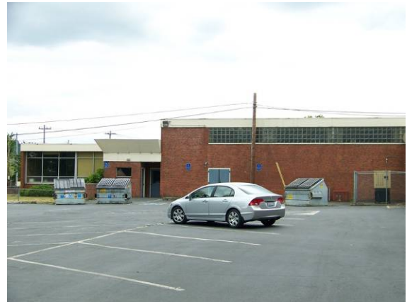
Main building (240A), north (side) elevation, looking south.
