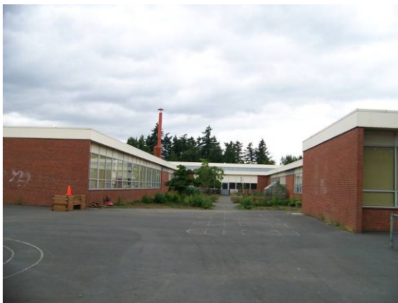
Main building (240A), south (side) elevations and courtyard, looking north.
