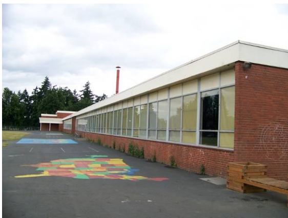
Main building (240A), west (side) elevation, looking north.
