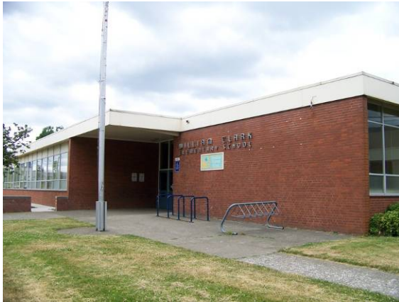
Main building (240A), east (front) and north (side) elevations, looking southwest.
