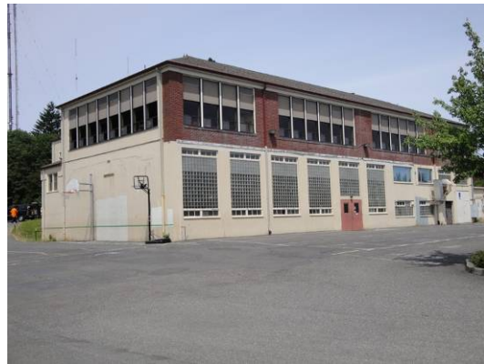
Gymnasium west and south elevations
