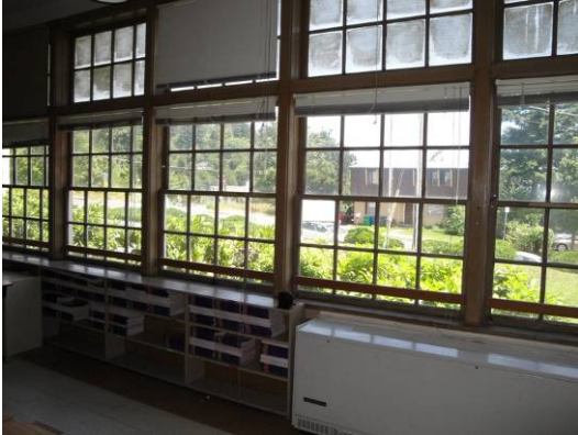
Main floor classroom facing east
