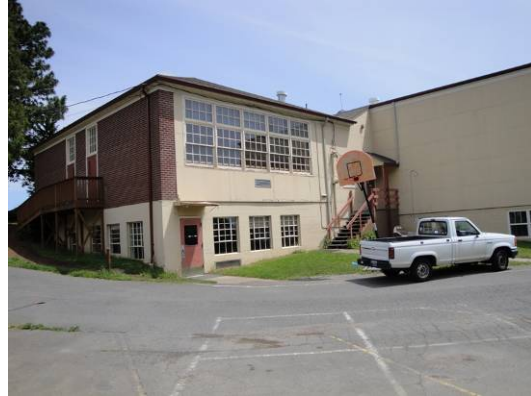
West (rear) and south elevations
