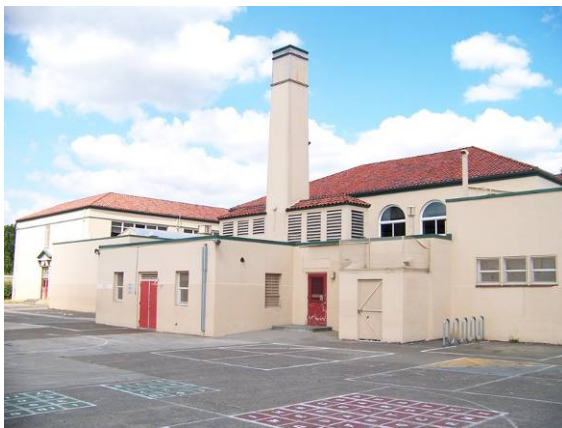
Main building (157A), west (rear) elevation, looking northeast.
