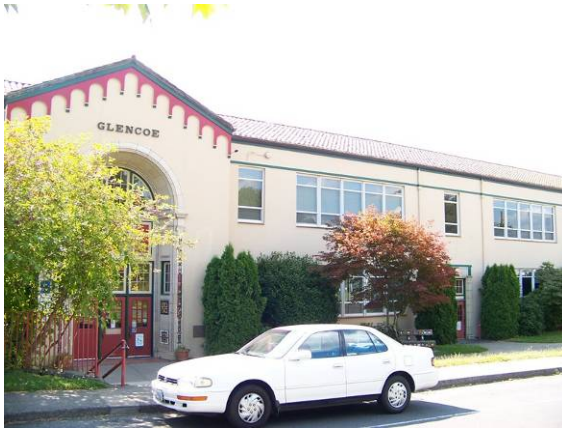
Main building (157A), east (front) elevation, looking northwest.
