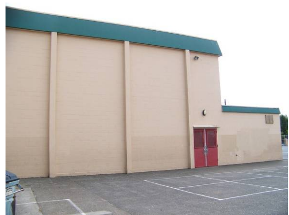
1964 addition, north elevation, looking southwest.
