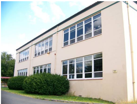
Main building (157A), north (side) elevation, looking southeast.
