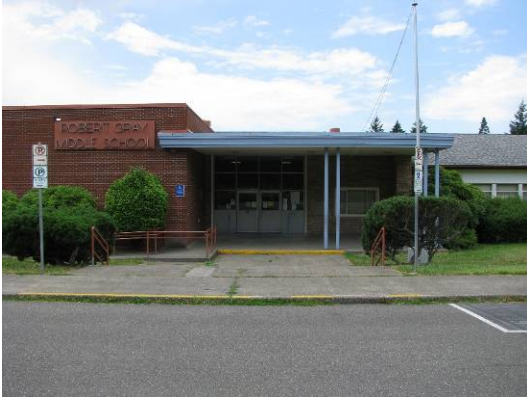
East elevation of main building (158A).
