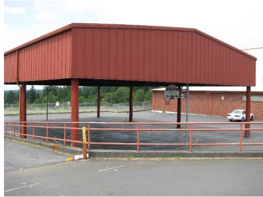
Play shed (158B), looking northwest.
