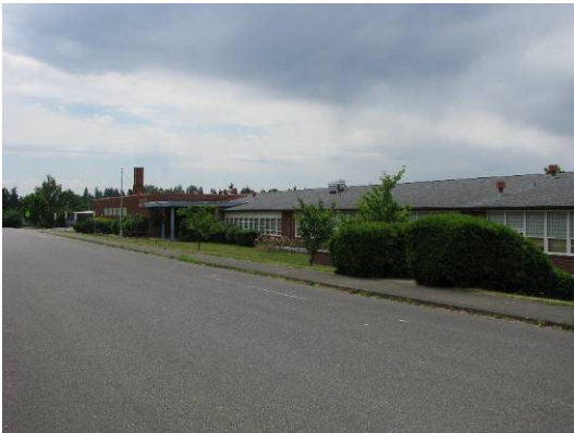
East elevation, main building, looking southwest (158A).
