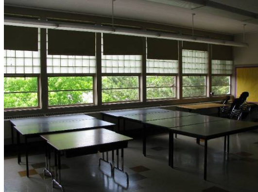
Typical classroom showing use of glass block (158A).
