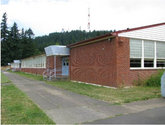
East elevation of main building (158A).
