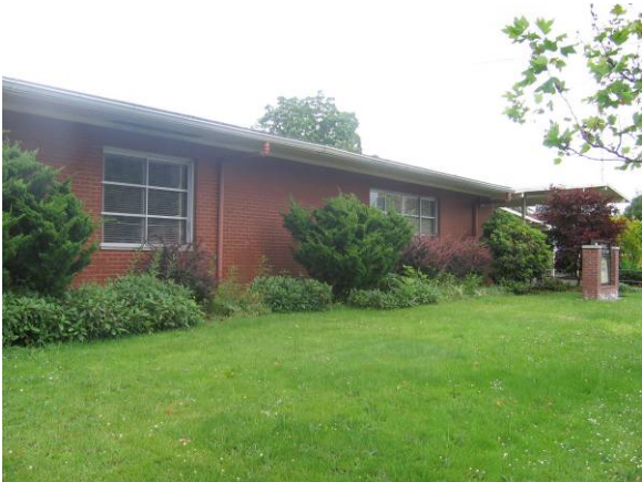
East elevation facing northwest
