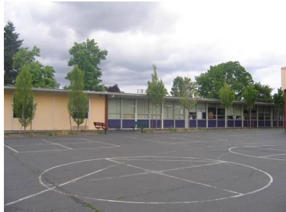
South elevation facing northwest
