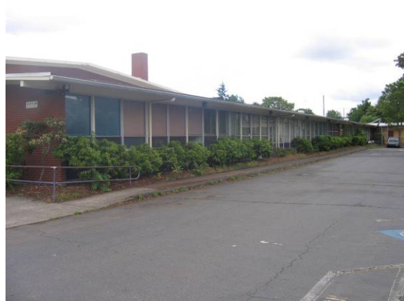
North elevation facing west
