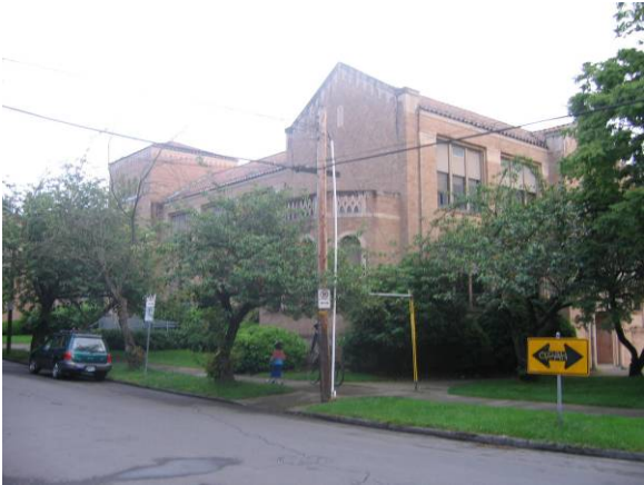
North elevation facing southeast
