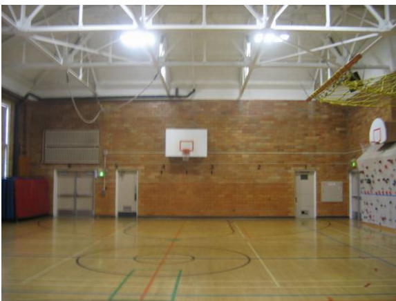
Gymnasium facing west
