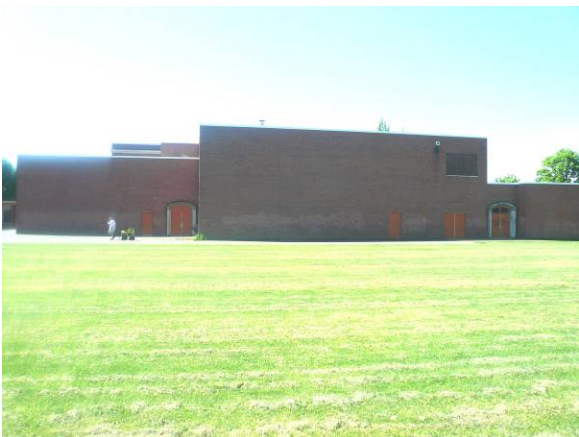
North elevation facing south
