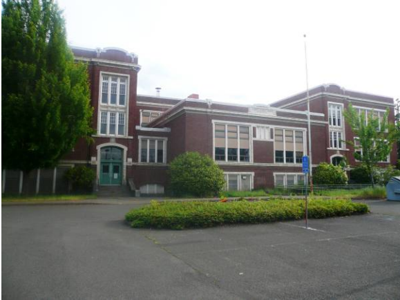
South elevation facing north
