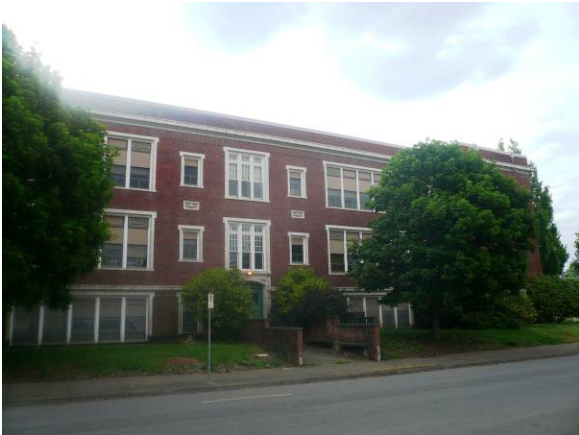
West elevation facing southwest
