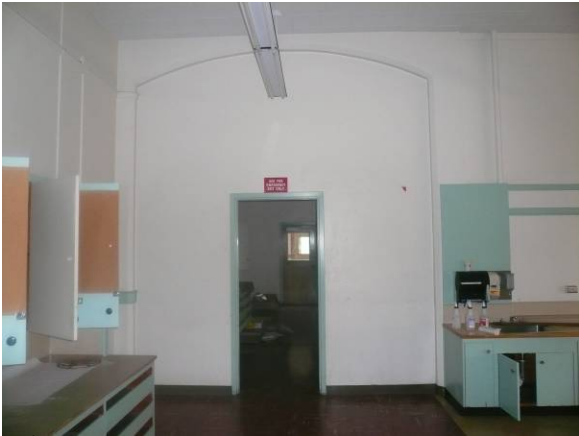
3 rd Floor corridor facing east
