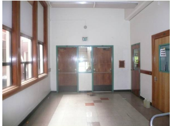
Corridor enclosed staircase and fire doors
