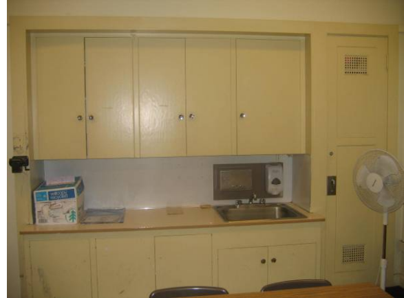
Classroom built-ins facing east
