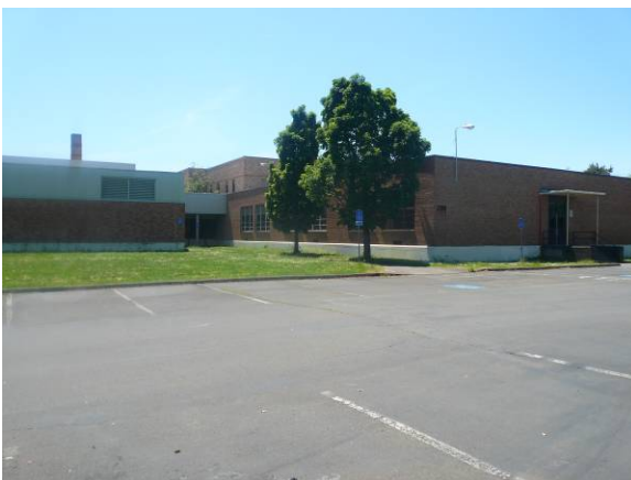
North elevation facing southeast
