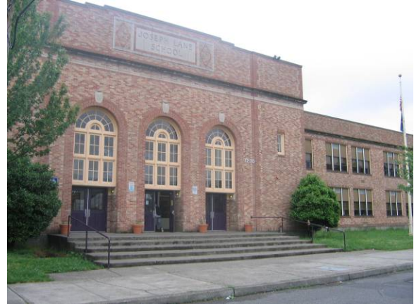
West elevation facing southeast
