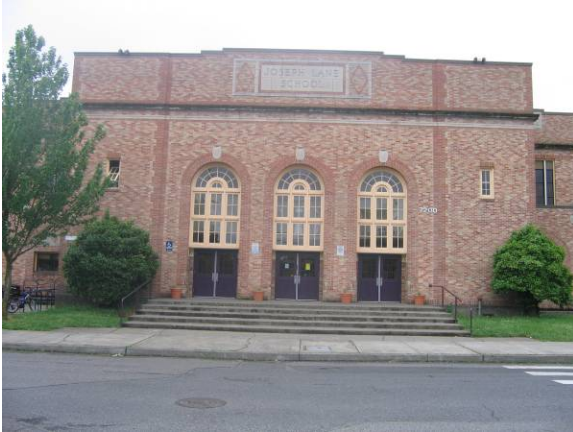
West elevation facing east
