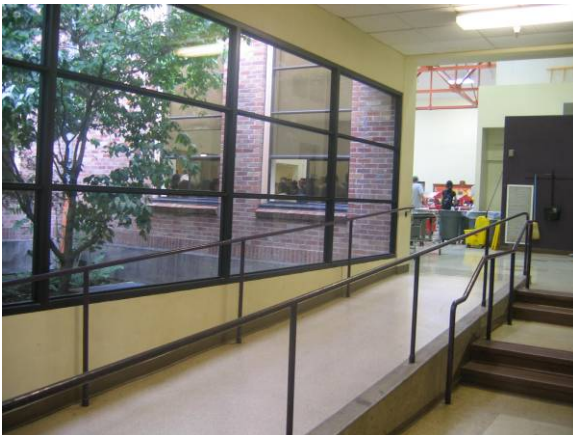
Ramp, staircase facing north
