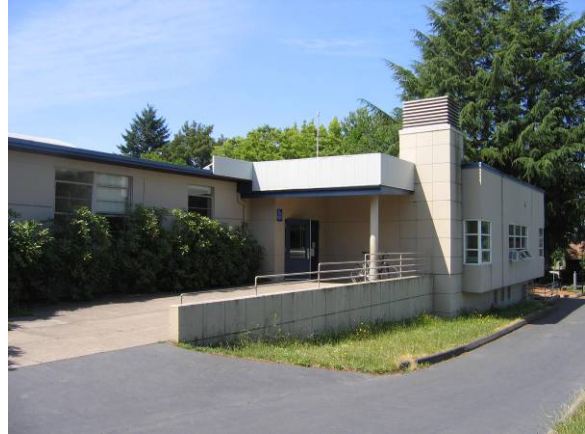
North elevation facing southeast
