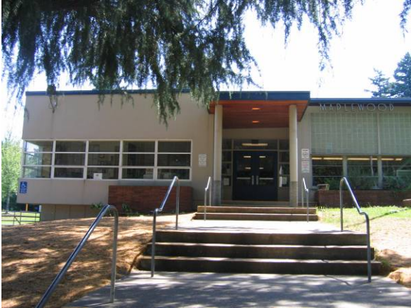
West elevation facing east
