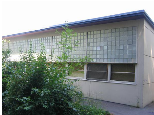
South elevation facing north
