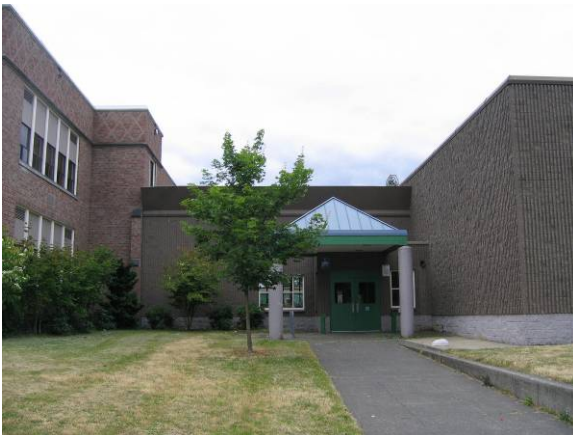
East elevation connection between main building and gymnasium
