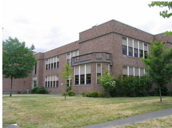
South elevation facing northwest
