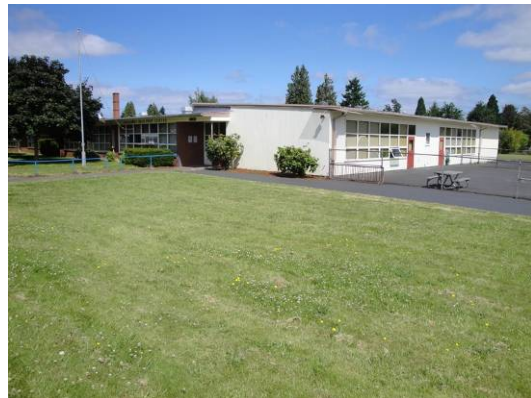
South and east elevations
