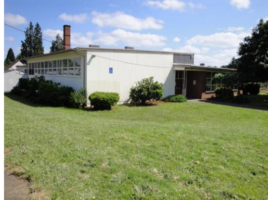
South (front) and west elevations
