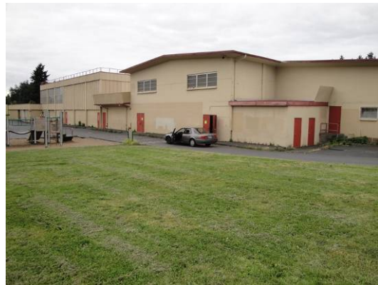
Gymnasium west elevation
