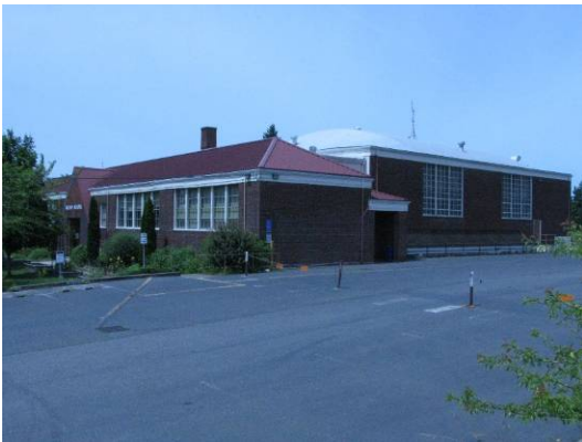
South and east elevations of main building (186A).
