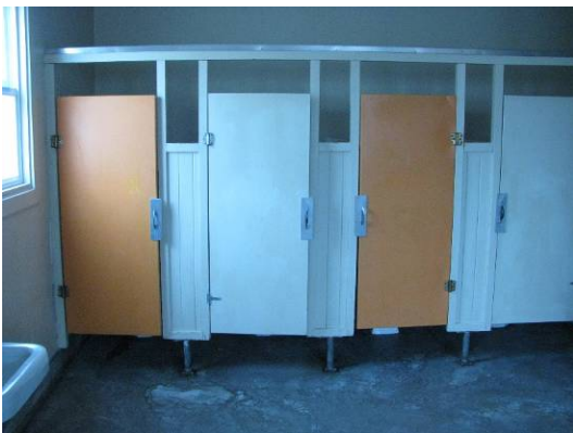
View of lavatory stalls (186A).
