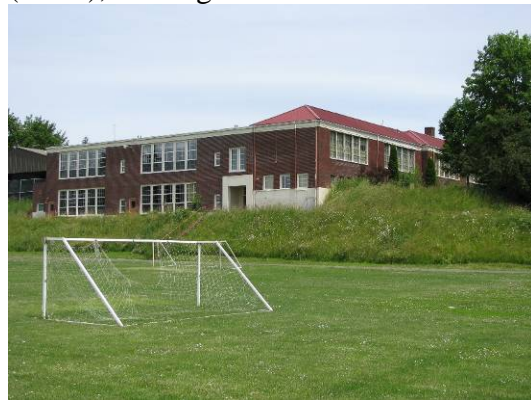
View of west and south elevations with view of 1956 addition.
