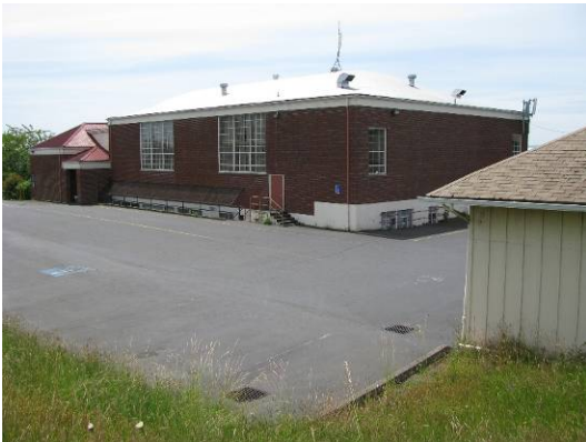
View of gymnasium (186A) looking southwest with garage in foreground (right).
