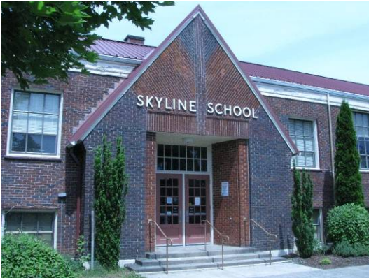
Main entrance, south elevation (186A).
