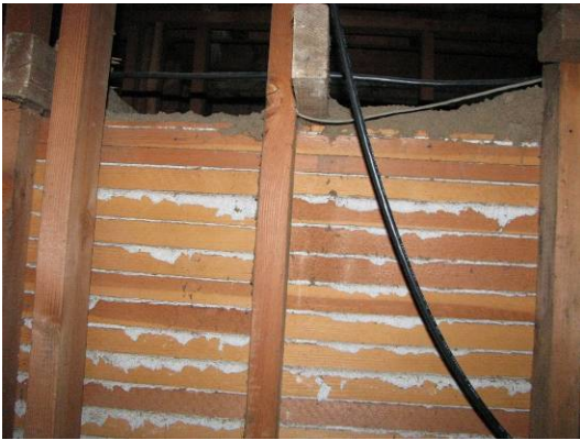
View of lath and plaster walls (186A).
