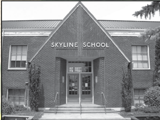
2009 photograph of west entrance into the Skyline School.
