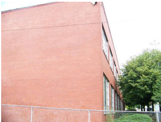
Main building (199A), east (side) elevation
