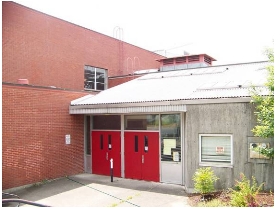
Main building (199A) and 1983 Entry Addition, north (side) and east (front) elevations
