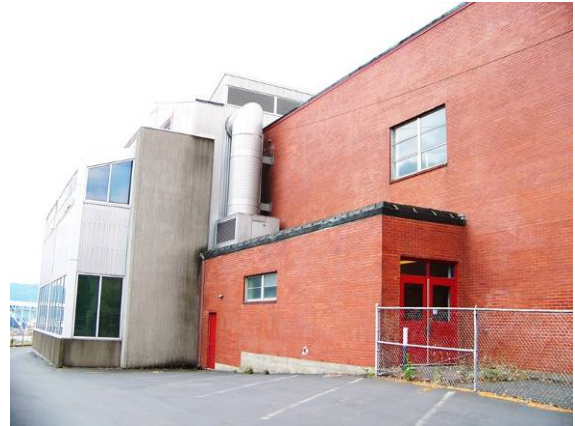
Main building (199A) and 1983 Addition (199B), south (side) elevation
