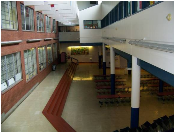
Main building (199A) and 1983 Addition (199B), commons area
