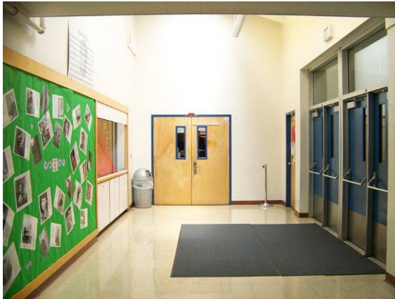
1983 Entrance Addition, foyer
