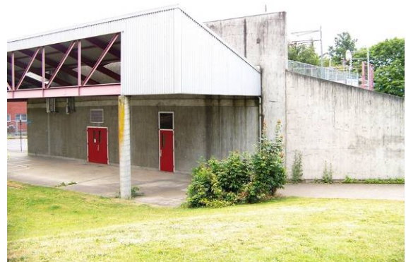
Industrial Arts building (199C), east (side) elevation and breezeway
