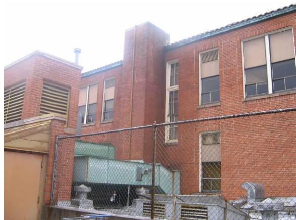
South elevation facing northwest
