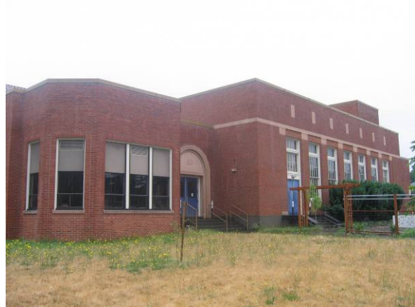
West elevation facing southeast
