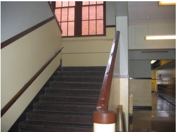
Staircase with handrail
