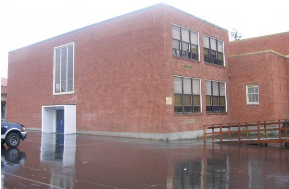
South elevation facing northwest
