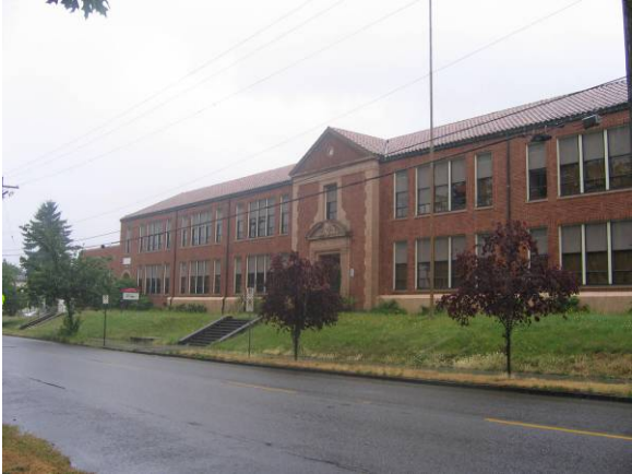
Entry facing northeast
