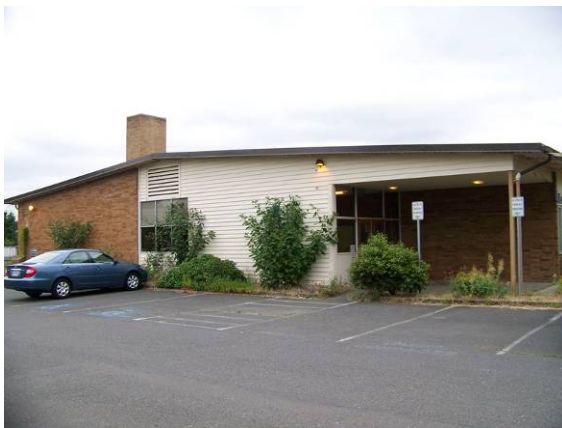
Main building (292A), south (side) elevation, looking north.
