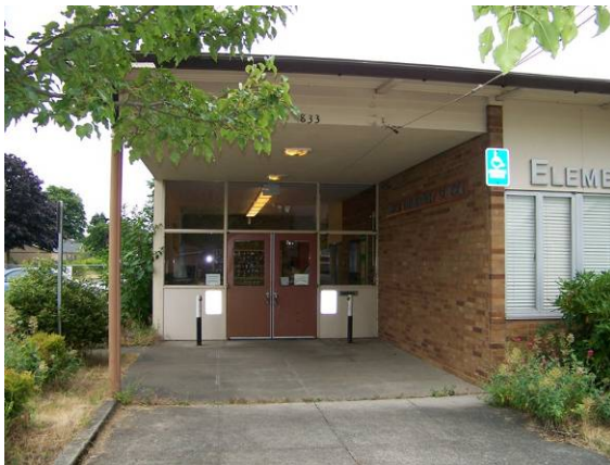
Main building (292A), entrance at east (front) elevation, looking west.
