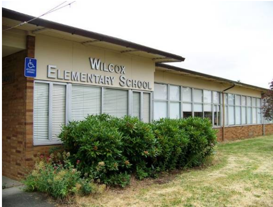
Main building (292A), east (front) elevation, looking northwest.
