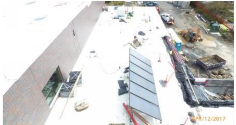
**Kitchen Roof – Solar PV Hot Water Panels Installed**
