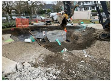
Installation of new storm system manhole on south March 2022 end of the site
