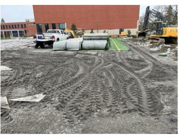
Rolls of removed artificial turf prepped for removal and recycling
