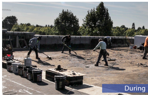
Complete roof replacement with seismic strengthening at roof level.
