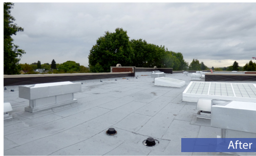
Complete roof replacement with seismic strengthening at roof level.
