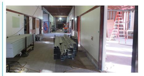
Area B2 seismic upgrades are wrapping up here soon. MEP/F system overhead rough-in is in progress with existing floor finishes in process. Interior wall framing is occurring on all floors. Fire rated ceiling metal framing followed by sheetrock is in process this month. The Area B2 Commons roofing is occurring this month followed along with installation of the MEP/F overhead rough-in. Many interior finish activities will begin to kick-off towards the end of this month.
