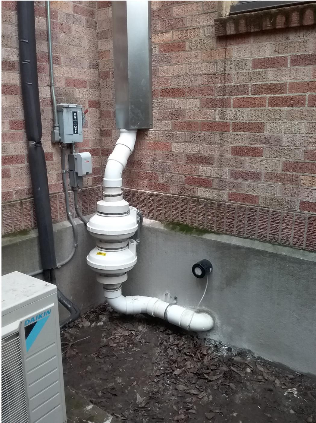
**The system includes an exterior rated manometer (pressure gauge), which is a simple means of seeing the system is working mechanically. A manometer also shows how much negative pressure (depressurization) the system is creating. It is understood such a pressure gauge DOES NOT monitor radon levels.**
