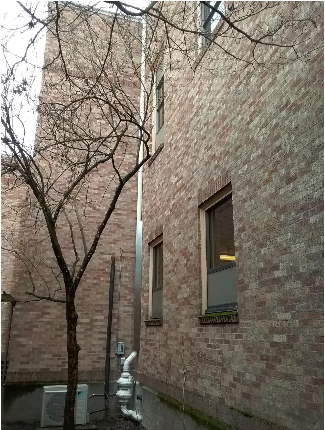
**A pipe shroud was installed to deter potential climbing on the vent piping running up the side of the building.**
